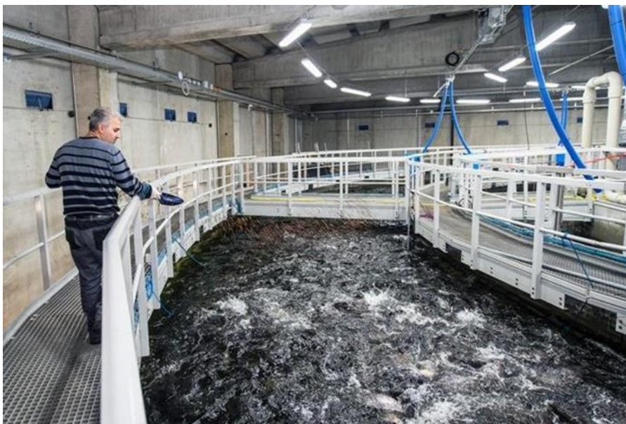
Figure 8: A large round tank (6 m deep, 32.5 m in diameter) as part of a salmon RAS (Swiss Alpine Fish)
