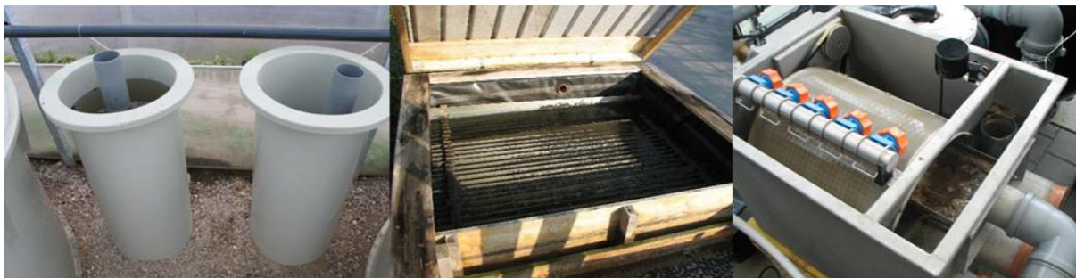
Figure 21: Different solids removal devices: (left) sludge trap; (centre) roughing filter; (right) rotational drum filter at ZHAW (all photos by U.Strniša)
